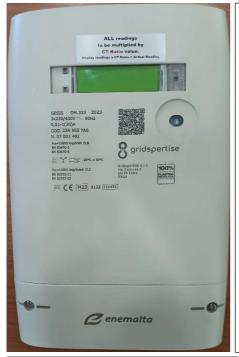
This is a new bulk supply meter used for 3 phase load currents that are greater than 60 Amp per phase.
